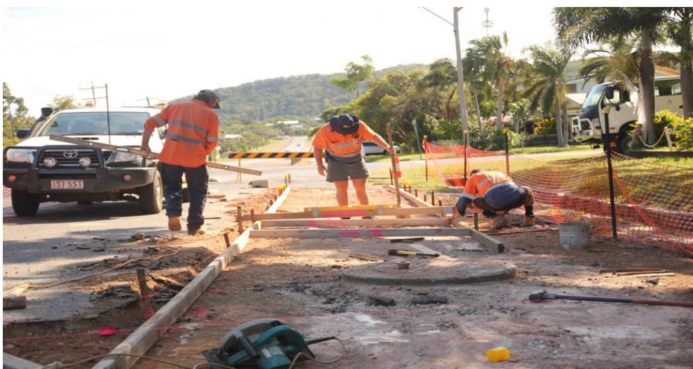
Footpath Construction Hope Street
