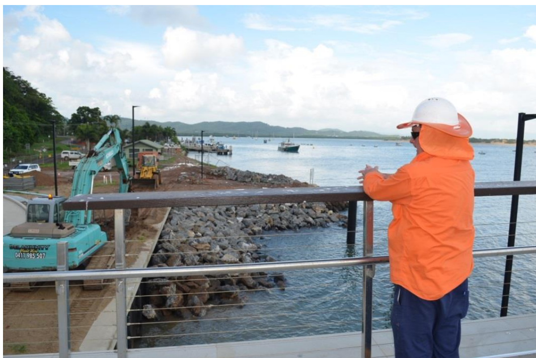
Cooktown Waterfront Construction
