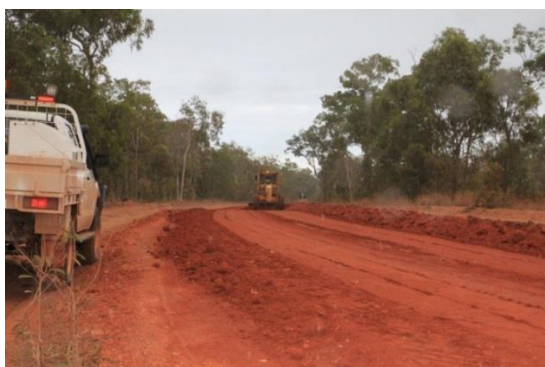
Roadworks at Lakefield National Park
